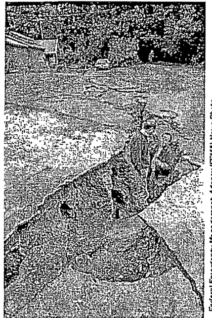
Fig. 2 These two men are standing in a roadway cut in half by the force of the Loma Prieta Earthquake on October 17, 1989.
