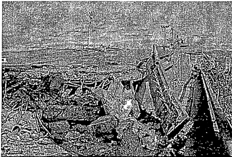
Fig. 1 Ground movement during the Loma Prieta Earthquake in California pancaked the upper deck of the Cypress Street Viaduct so that the guardrail seen on the right dropped to the lower deck.
